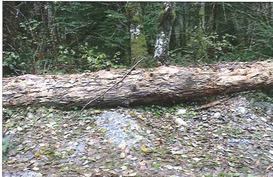
CK2263 Broken Stringer that was removed
